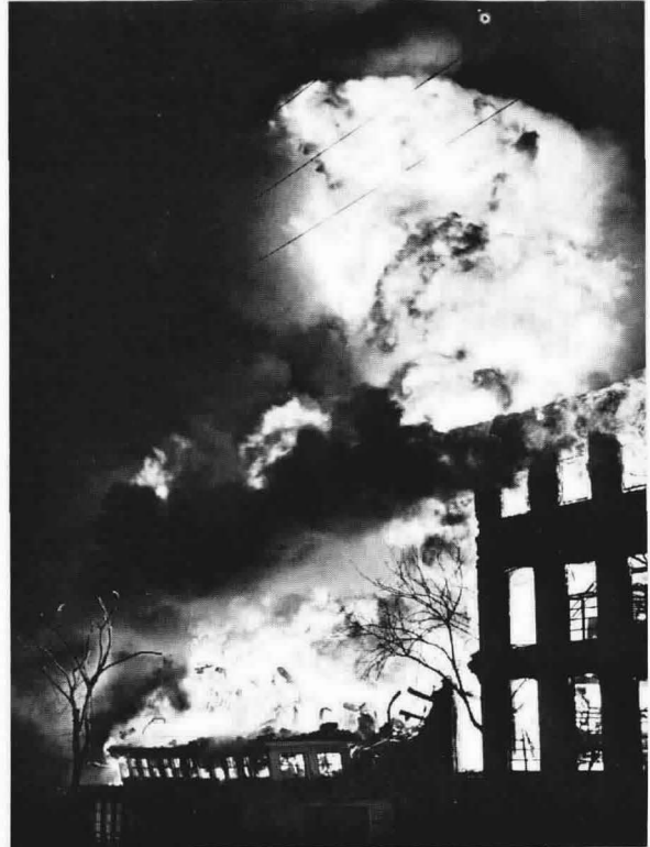
Above: Fairgrounds exhibition building fire of September 7, 1960, in Springfield, Missouri. The 12- to 20-foot-high wooden building with stone walls contained wooden bleachers and dry tanbark on the floor. The concentration of combustibles led to a huge fire in the isolated location, spreading to barns 30 to 60 feet away. This photo illustrates the difficulty in determining the exact height of flames when there is reflection from smoke rising from the fire. The flames, however, did extend much higher than in the average fire considered in this study.
