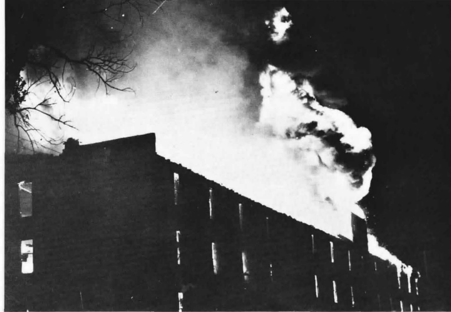
Left: Electrical appliance assembly building fire of May 19, 1965, in Hannibal, Missouri. The fire started in the second story of the four-story building of ordinary construction and involved the upper three stories. The sudden burst of flame at the right of the picture was probably caused by the release of flammable liquids. For most of the roof area the flames do not extend much more than 20 feet high. The building is 45 feet high.
