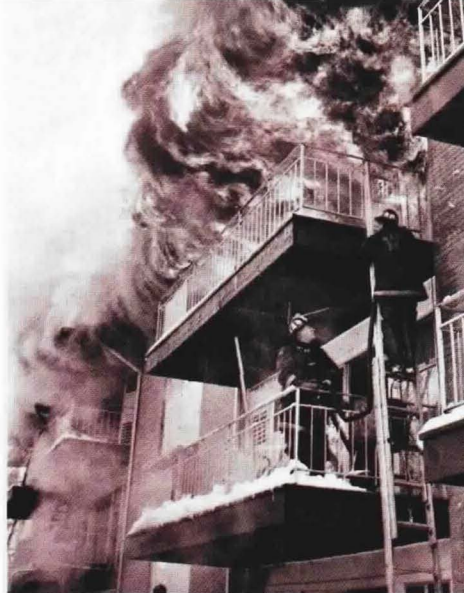
Figure 4. Flames billowing from apartment of fire origin. Note that there is no area of refuge on these balconies for occupants awaiting rescue.
