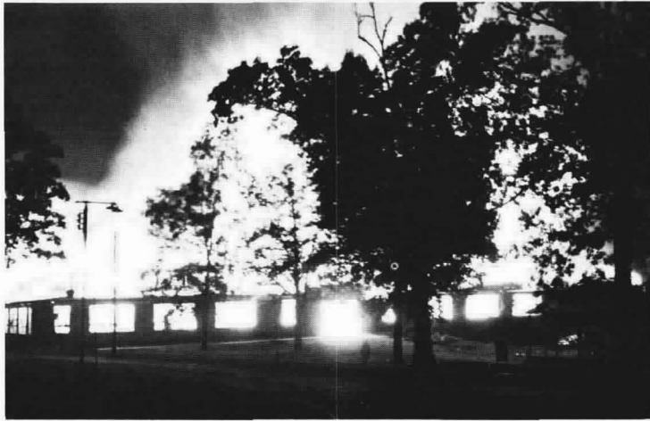
Above: Fairgrounds exhibition building fire of September 7, 1960, in Springfield, Missouri. The 12- to 20-foot-high wooden building with stone walls contained wooden bleachers and dry tanbark on the floor. The concentration of combustibles led to a huge fire in the isolated location, spreading to barns 30 to 60 feet away. This photo illustrates the difficulty in determining the exact height of flames when there is reflection from smoke rising from the fire. The flames, however, did extend much higher than in the average fire considered in this study.
