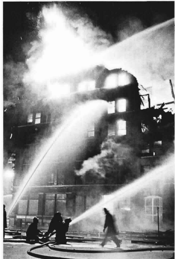
Right: Woonsocket, Rhode Island, April 29, 1967. A four-story (50-foot-high) worsted mill ablaze on all four sides, with the flames from the roof equivalent in height to more than three stories. The plant was of mill construction and processed both wool and synthetic yarns. The fire, which started in the first floor from malicious use of gasoline, resulted in rapid spread of flames that overpowered the sprinkler system. Because the vertical cutoffs were incomplete, the fire soon spread to the upper stories. By the time the picture was taken, the first story had been practically burned out.
