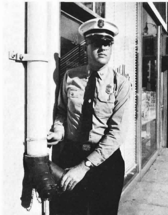
An inspector examines a new standpipe where the old standpipe had failed completely. The old standpipe, encased in the brick veneer of the building, ruptured in the pressure test. The building management decided that it would be less expensive to install a new standpipe than to remove the brick façade and repair the old pipe.
