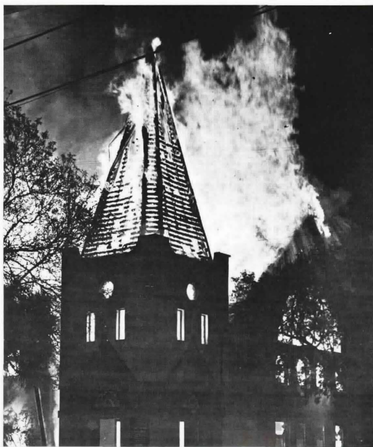
Right: Church fire of December 13, 1960, in Palo Alto, California. The church, of ordinary construction, was the equivalent of a three-story building in height. The chief combustibles present were the wooden pews, flooring, and roof, but the flames extended at least two stories above the roof.
