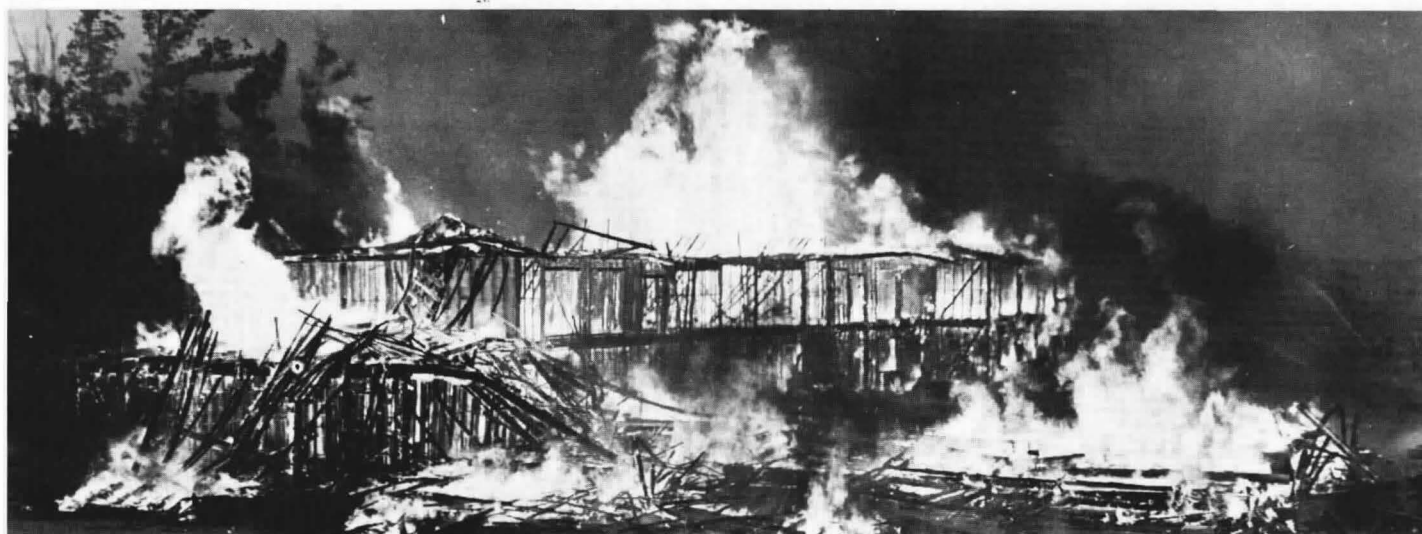
Above: This two-story apartment house of wooden construction in Hampton, Virginia, had not quite been completed when a fire of undetermined cause destroyed it on August 25, 1965. High wind and lack of nearby hydrants were factors. The flames extended the equivalent of two or two and a half stories above the roof line.
