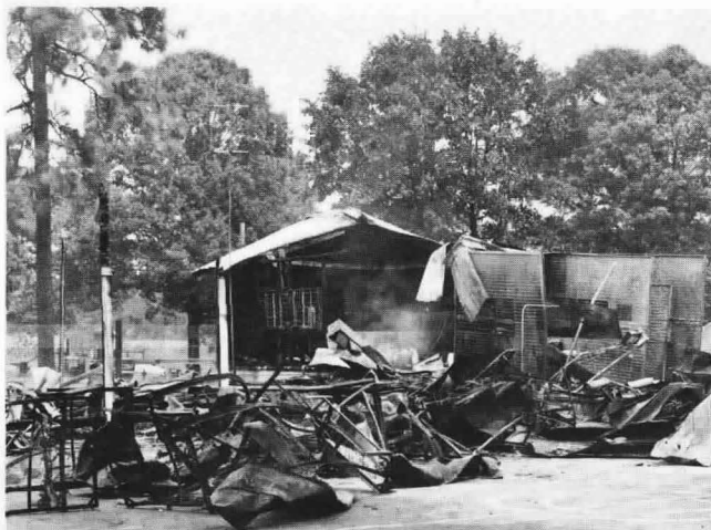
A fire started by prisoners during a riot quickly consumed this wooden prison barracks in Berrydale, Florida, leaving 38 prisoners dead — the largest loss of life in a single fire in the United States or Canada in 1967. The metal cage in the foreground was the guard station.
